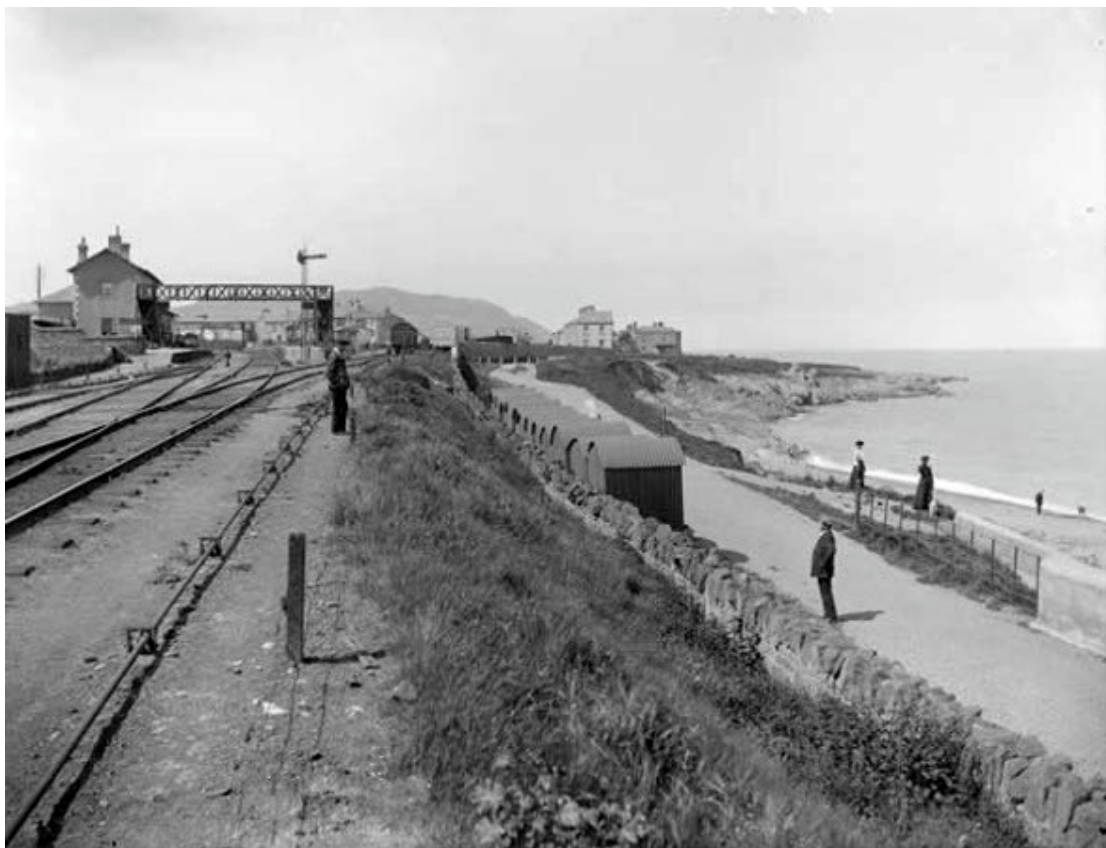
Greystones railway station and beach, 1880 - 1914
