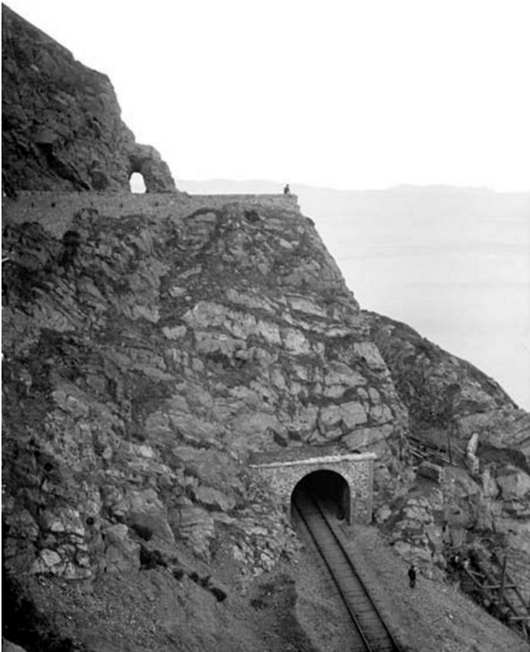
Bray Head Tunnel
