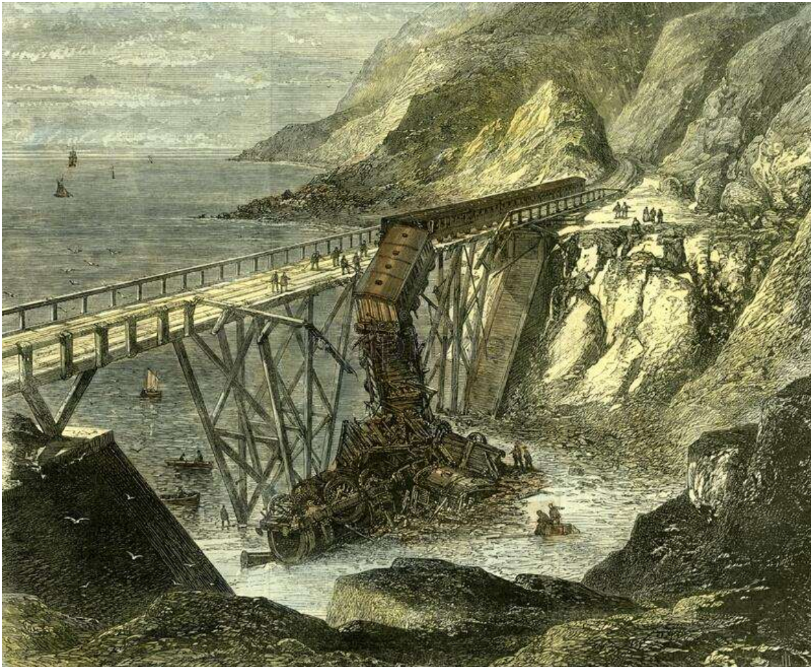
Railway accident at Bray Head, 1867
