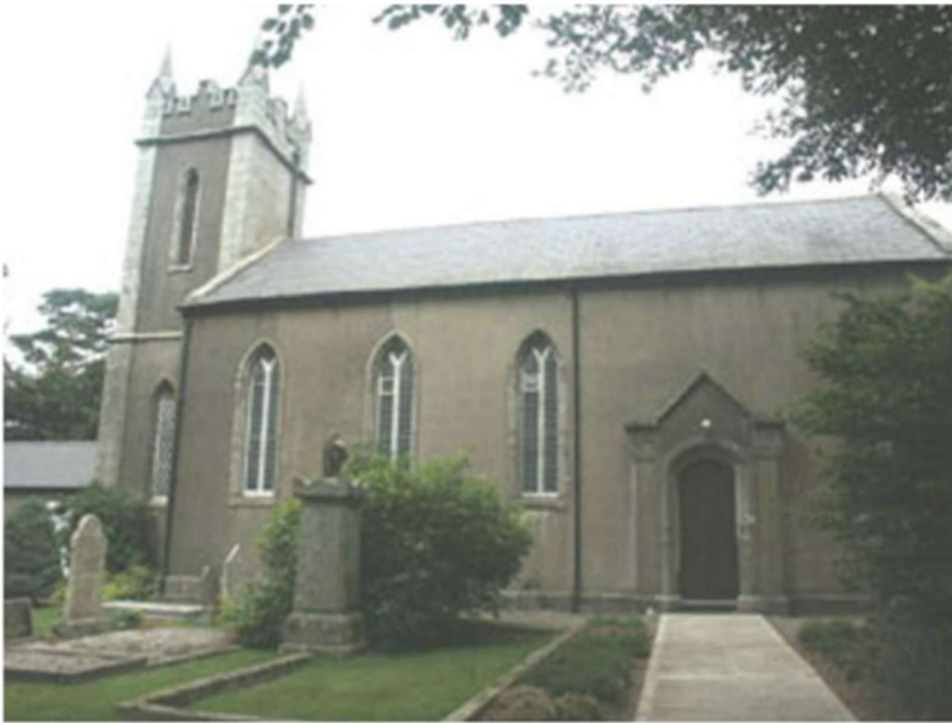
Calary Church (National Inventory of Architectural Heritage)
