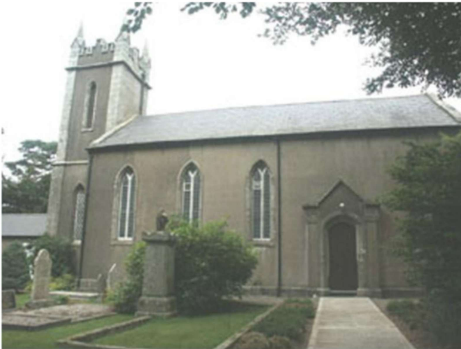
Calary Church (National Inventory of Architectural Heritage)
